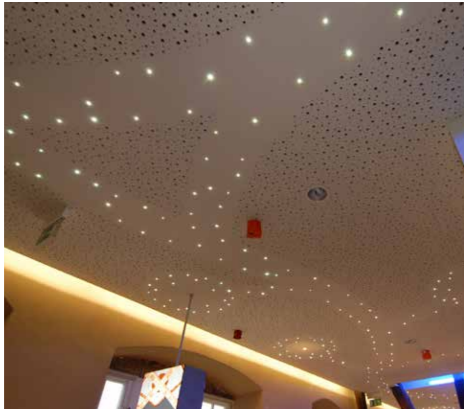
VoglJoint panels according to layout plan
