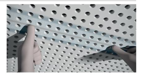
Apply another generous layer of Liquid Glue over the tape with the roller, applying slight pressure as you roll.
