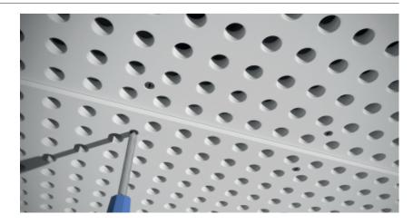
Provide an expansion joint of 5 - 10mm every 100m<sup>2</sup> or 10 lineal meters.
