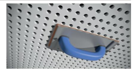
Slightly dampen joint area using a sponge, but avoid excessive wetting of Vogl panels.
