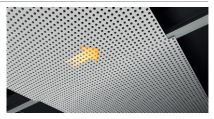
Fix the screws in the panel joint in alternating patterns (zig-zag method) on the left and right side of the locating screw. This will create a tight and flush joint and ensure it is evenly aligned.
