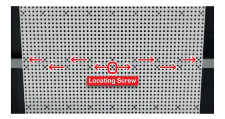
Install ceiling panels first lengthways, then crossways, resulting in cross arrangement on ceiling. Cover remaining areas in same manner, working from centre of room outwards.
