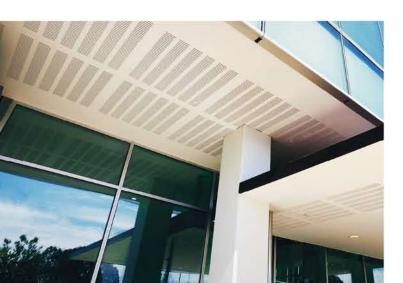
Au.diVent slotted fibre cement panels are the slotted alternative to Au.diLux panels. Ideal as acoustic control panels or as ventilation panels, directing heat and moist air outside to prevent condensation build-up in roof cavities.
