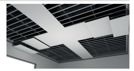
After all panels have been installed, re-check that all joints are level and adjust, if necessary, using a screwdriver. Then check with a straightedge.
