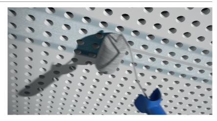
Do not clean or scrape the joint when it is wet as it will damage the tape and joint system.
