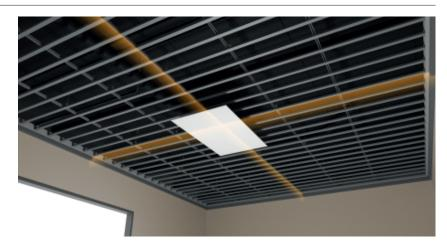
Insert the supplied screws at right angles, direct in to the furring channel, and counter sink to 0.5mm below the panel surface.
