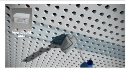
Whilst the glue is still wet, apply the supplied 8mm joint tape over the panel joint, ensuring the shiny, rubber side of the tape is facing the ceiling panels.
